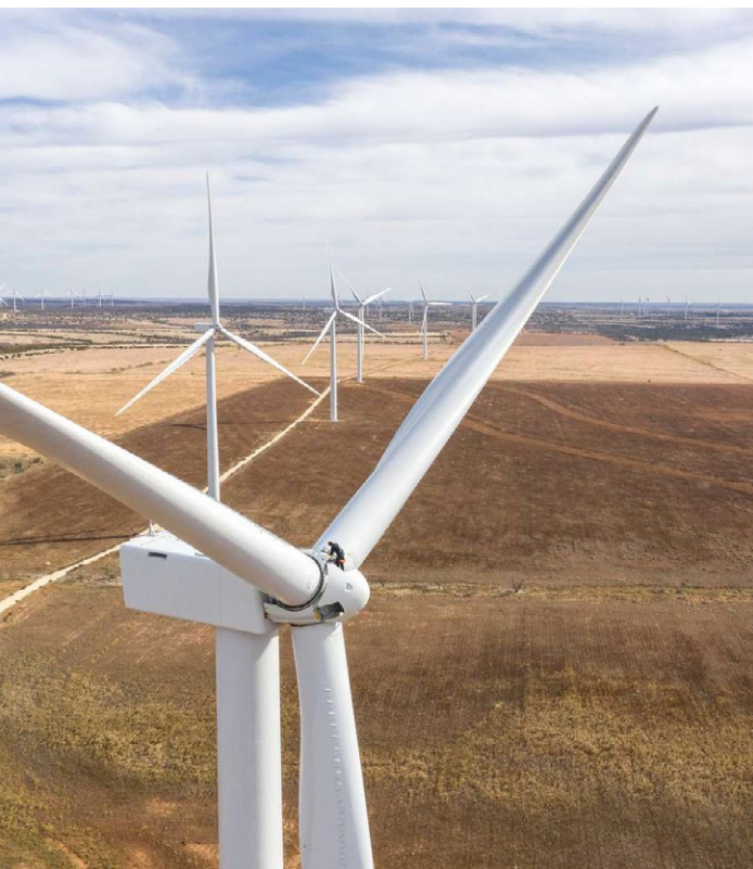
Amazon Wind Farm, Scurry County, Texas, the US.
