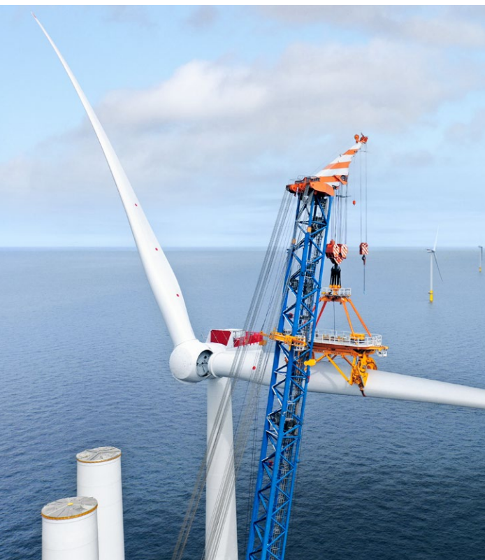
Installation of blades at Hornsea 2, the UK.
