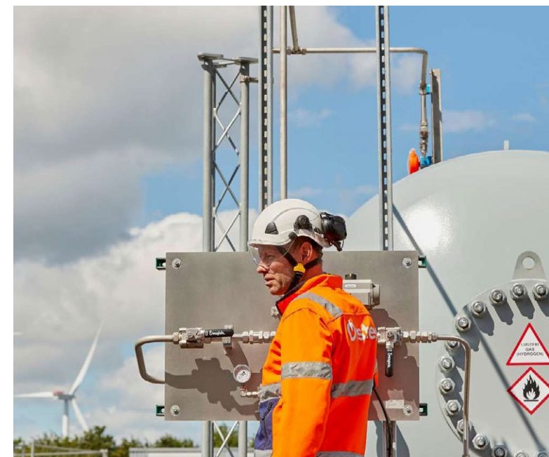
Our hydrogen test facility at Avedøre Power Station, Copenhagen, Denmark.
