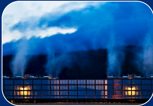
Data Center Heat Recovery
