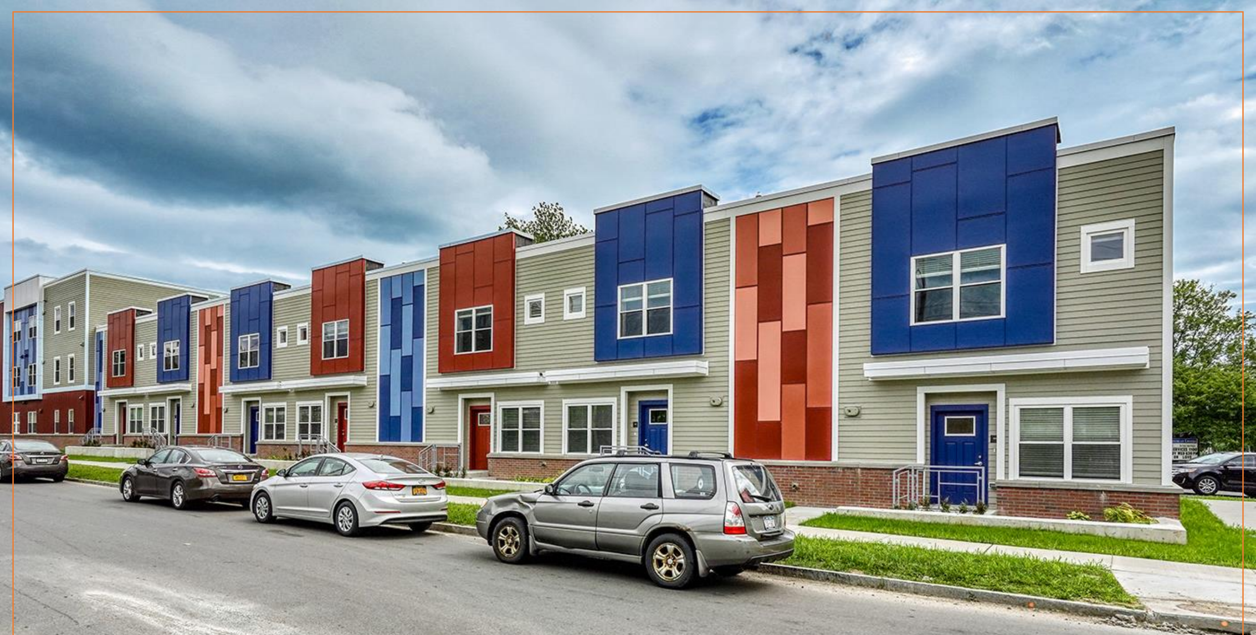
Freedom Commons – LEED Gold Certified 2019; SHA’s commitment to building green.
