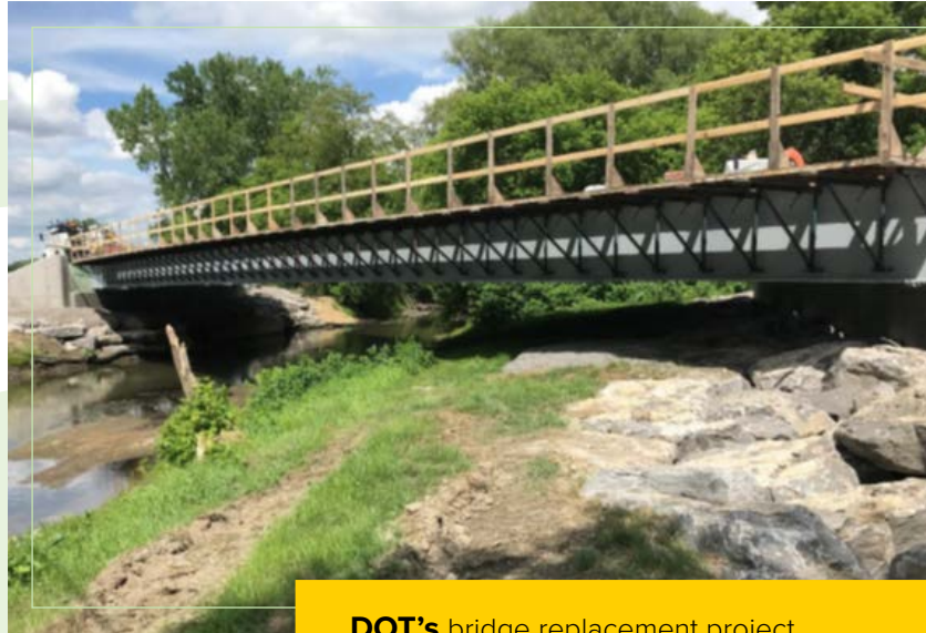
DOT's bridge replacement project on Route 19 over Oatka Creek.
