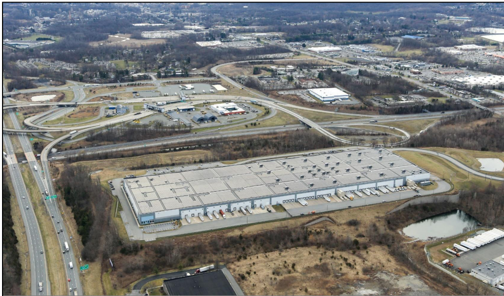
PV on Newburgh distribution center
