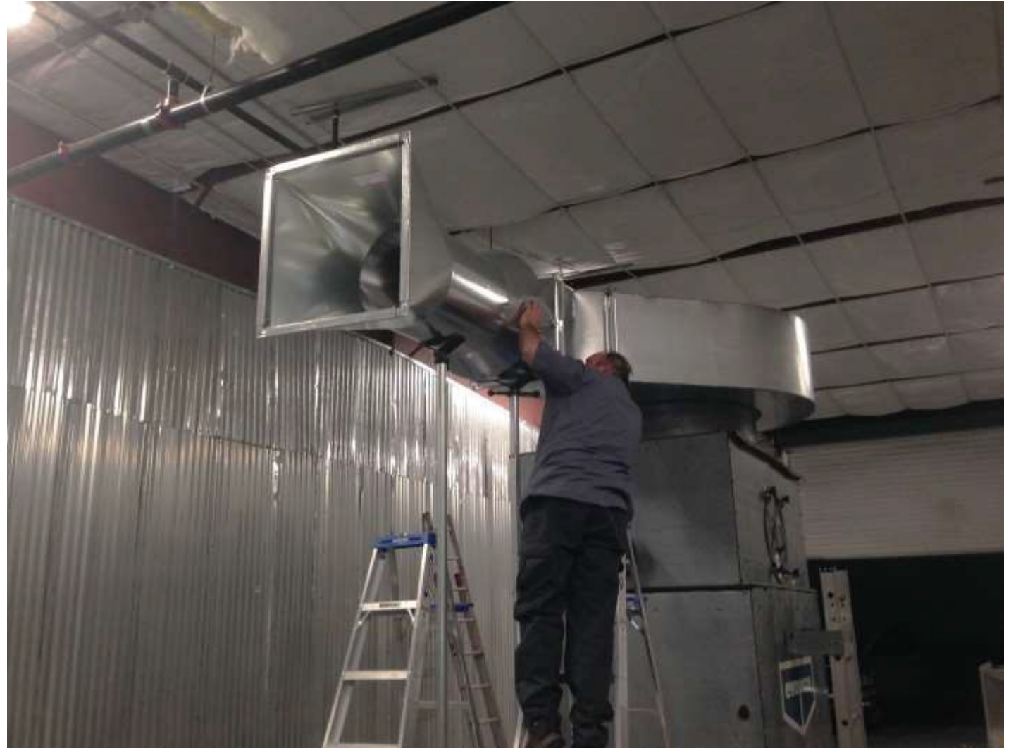
Rob Allison installing early prototype
