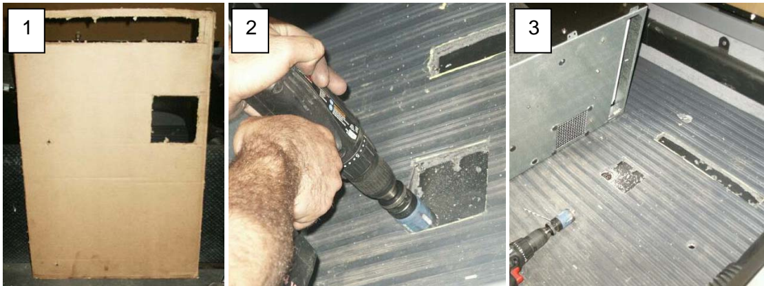
Figure 5: Template and cutting of HVAC drain and air discharge holes
