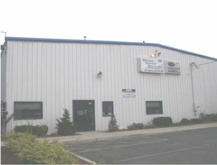
Figure 2. NTR Installation Facility in Albany, New York
