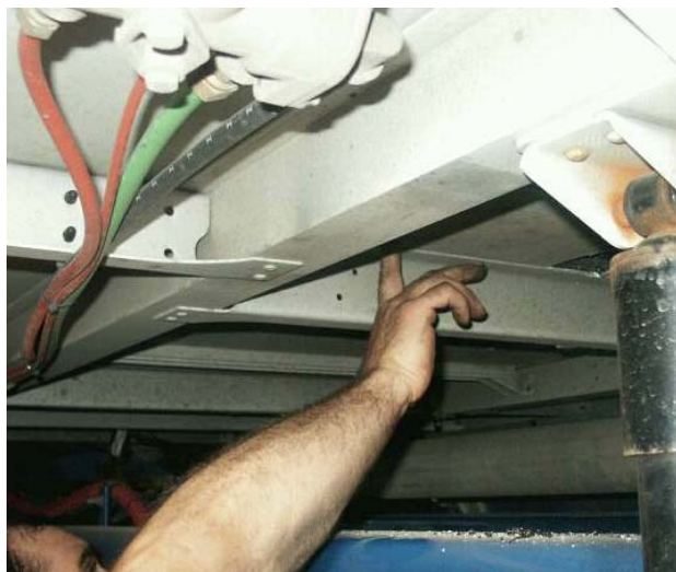
Figure 3: Underbody inspection for HVAC location selection
