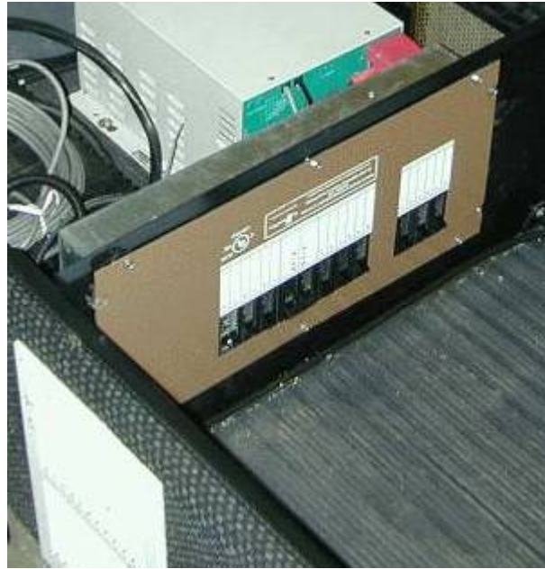
Figure 22: Completed installation of the Intellitec distribution panel
