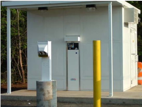
Figure 7. Pedestal and Utility Building
