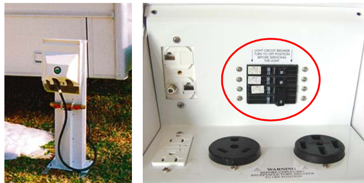
Figure 6. Lift cover to view breakers and outlets. Always turn breakers to the OFF position before plugging in or removing any plugs
