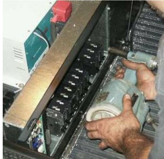
Figure 17: Mounting the Intellitec distribution panel
