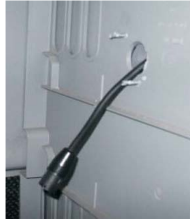
Figure 24: Inside of cabinet for electrical outlet mounting
