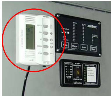
Figure 8. Cab Comfort HVAC remote/ display mounted behind the clothes/ TV cabinet
