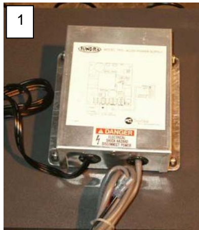
Figure 42: 12VDC-120VAC refrigerator inverter installation
