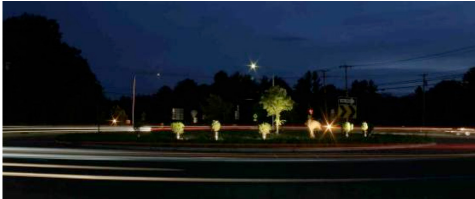
Figure 33. Vegetation and landscape lighting installed at a roundabout
