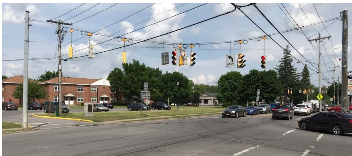
Figure 7. Intersection of Leland Avenue and NYS Route 5
