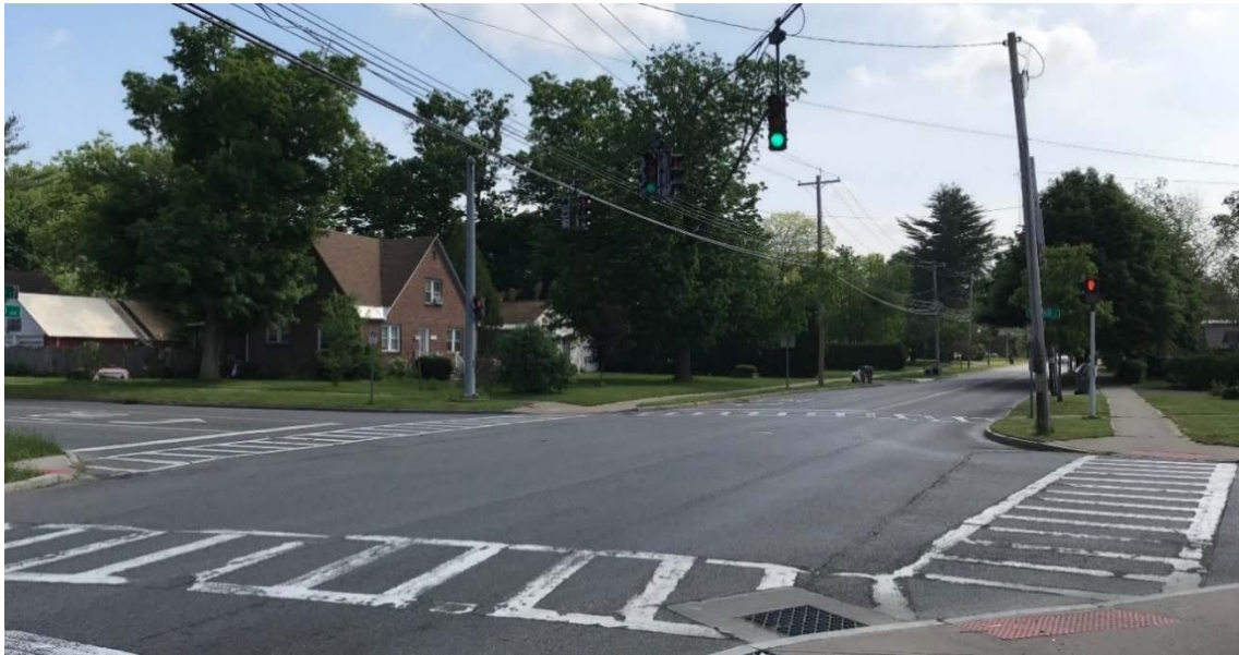
Figure 11. Intersection of Floyd Avenue and Oakwood Street
