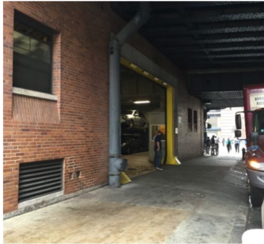
Conditions under the viaduct vary
