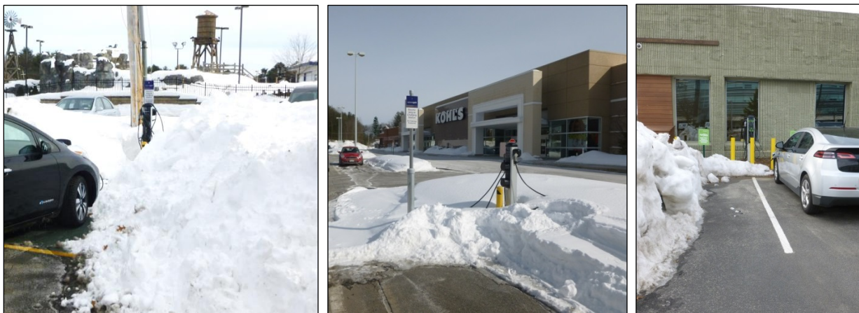
Figure 19: Snow management practices may impede EV charging
