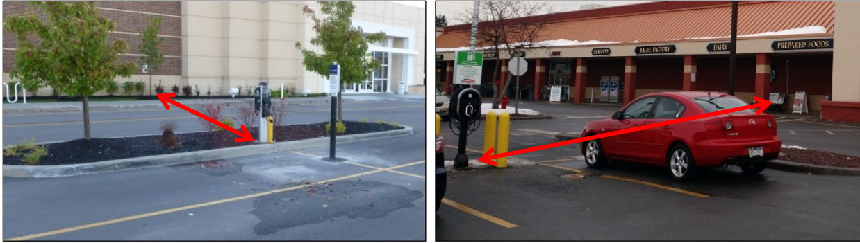
Figure 14: Charging stations at parking spaces away from a building require longer trenching through pavement and could disrupt traffic flow during construction
