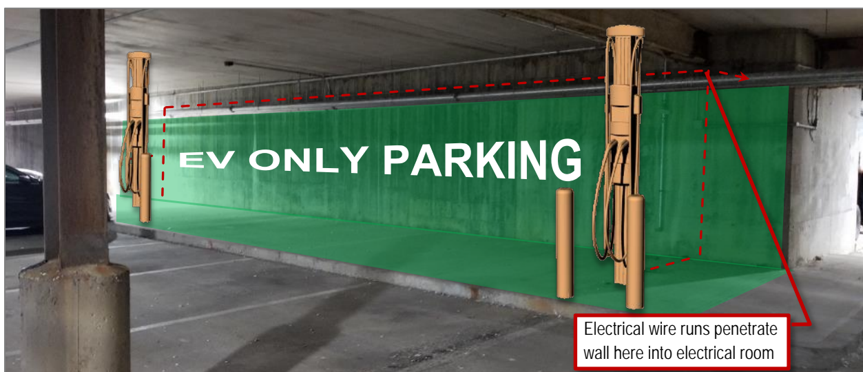
Figure 9. First potential EV charging location in Barnes and Nobles employee parking garage
