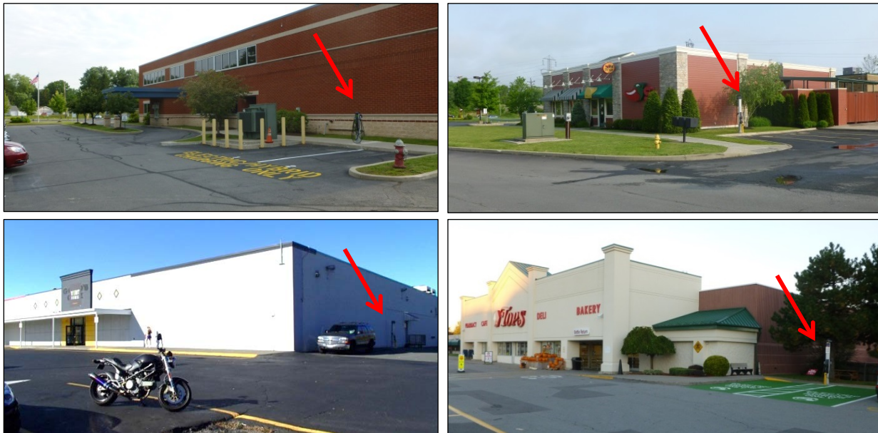
Figure 13: Charging station installations sited in convenient, but not prime parking spaces that minimize conduit runs to reduce costs
