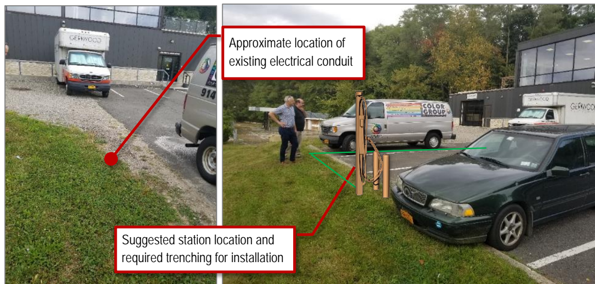
Figure 16. Potential EV charging station installation location at Candela Lighting Systems
