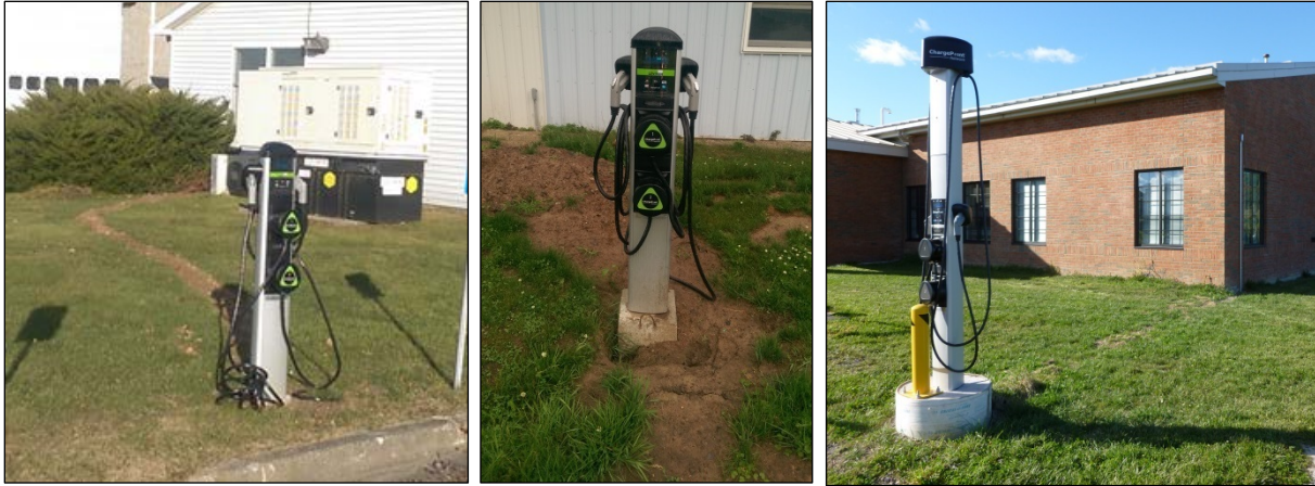
Figure 16: Examples of trenching through dirt (easiest outdoor installations)
