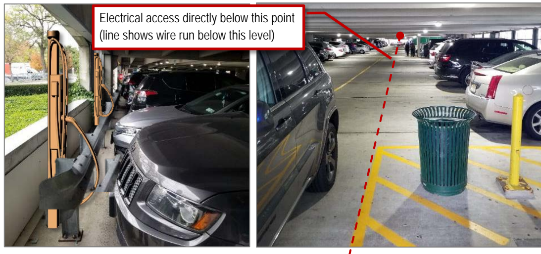
Figure 19. Potential EV charging station installation location at Fordham University Parking Garage
