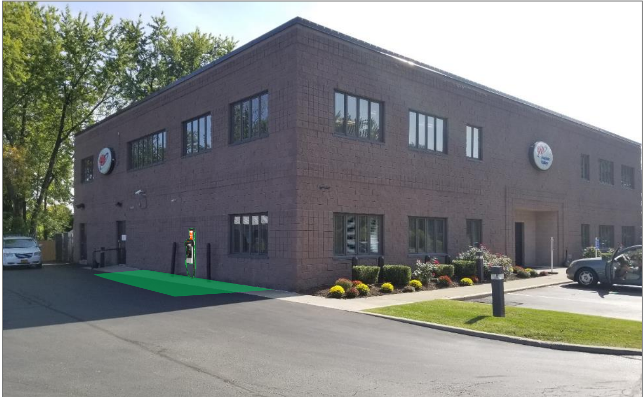
Figure 21. Potential EV charging station installation location at AAA Hudson Valley
