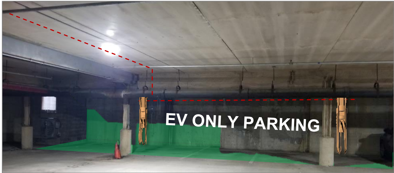
Figure 10. Second potential EV charging location in Barnes and Nobles employee parking garage
