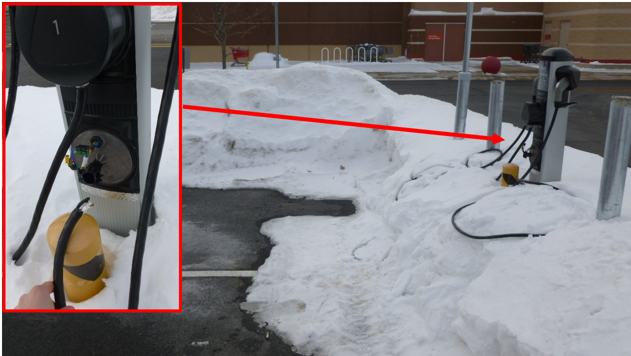
Figure 20. Charging cords not coiled up in the winter can be covered with snow and caught by a plow
