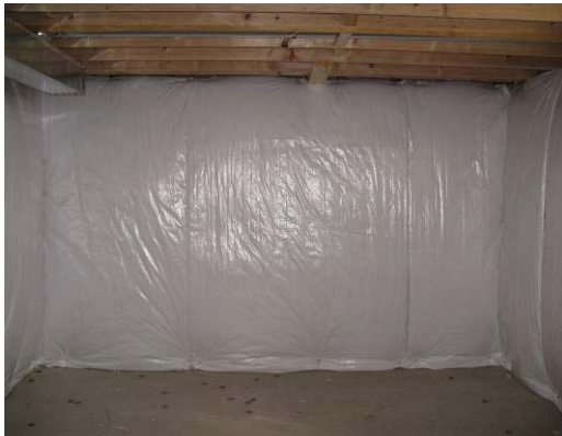
R-26 blanket insulation installed in basement
