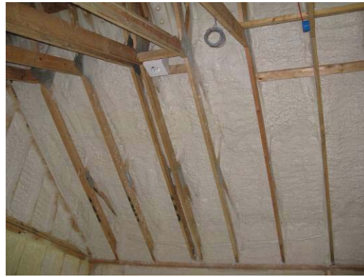
Ceiling after application of spray foam
