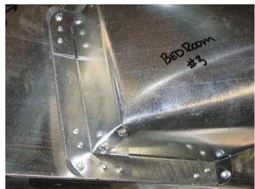
Branch elbow, after attachment to the ventilation trunk
