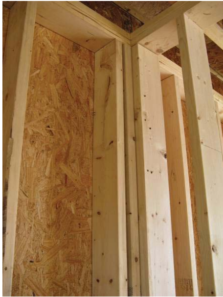
One corner in the home with five studs next each other
