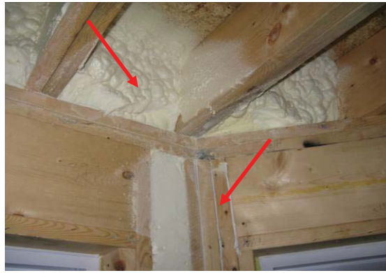
Spray foam in rim joists and tight corner, and caulk sealing gaps in framing members
