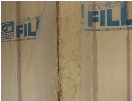
Exterior walls – “flash and batt” method
