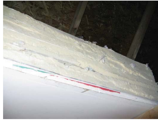
Attic hatch with four layers of insulation foam board
