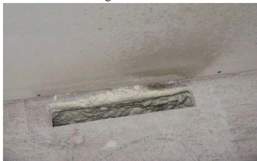
Sealed duct work and sprayed around section – great work
