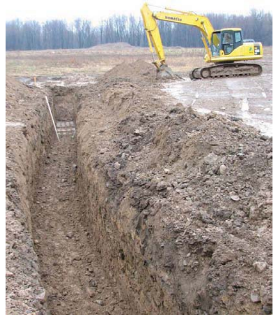
Excavating for the horizontal geothermal loop field
