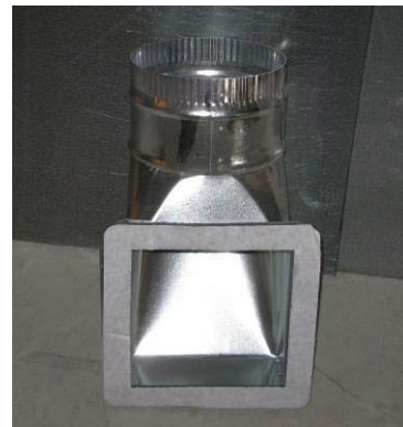
Branch elbow before being attached
