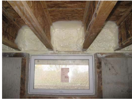
Replacement spray foam that has properly expanded
