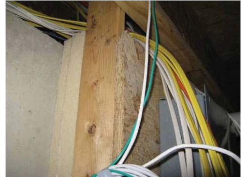
Insulation foam board behind the electrical panel.
