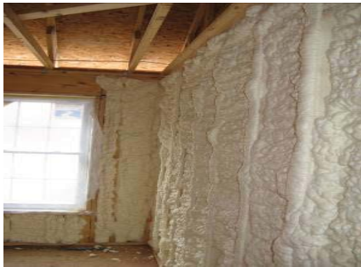
Wall cavities filled with spray foam before being trimmed
