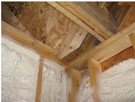
Tight corner at intersection of house and garage roof lines
