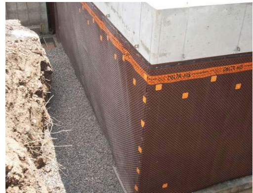
Below grade walls’ moisture membrane before backfill
