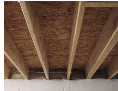
First floor joist system
