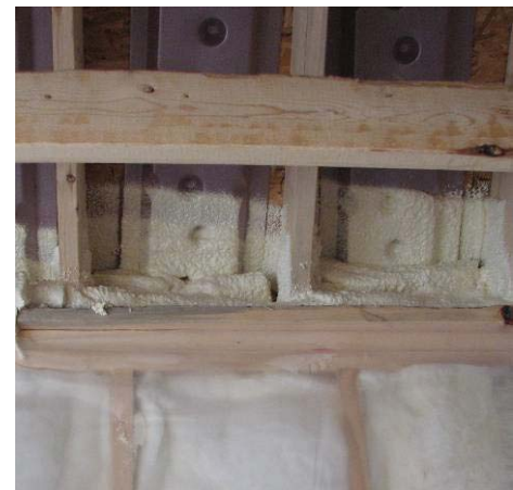
Overhang sealed with spray foam
