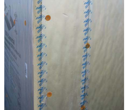
Exterior insulation with cap nails and seam tape
