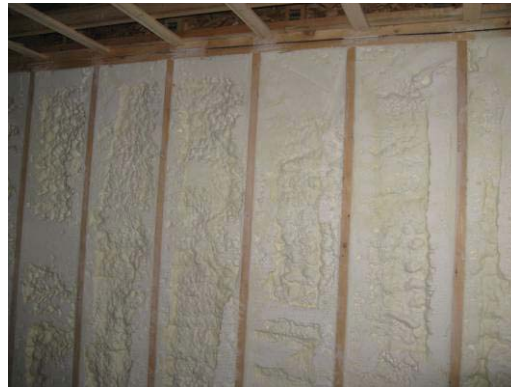
Wall cavities filled with spray foam that has been trimmed
