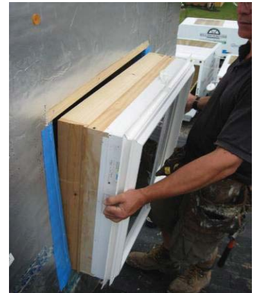
Window is set flush against the sealant. Note the extended jambs
