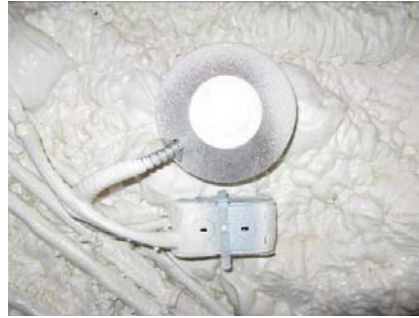
Recessed lights after spray foam was applied from inside the attic
