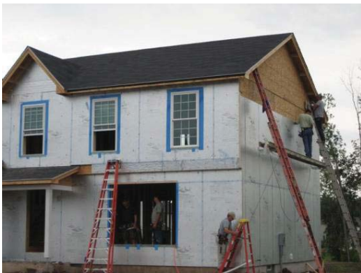
Exterior insulation being installed by the window installation contractor
