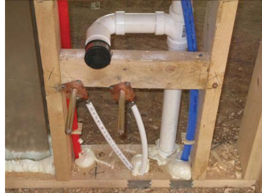
Sealing with expanding foam
