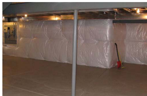
Basement Walls: R-25 fiberglass insulation blanket with perforated FSK facing
