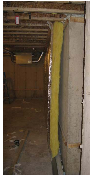
Full length blanket insulation being installed on below grade wall.
