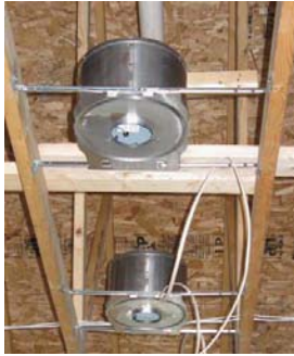
Enclosed recessed lights before spray foam application from the ground
