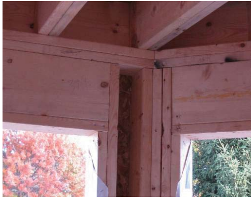
Spray foam in rim joists and tight corner, and caulk sealing gaps in framing members
