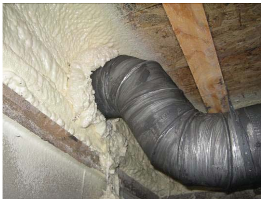
Sealed duct work and sprayed around section – great work
