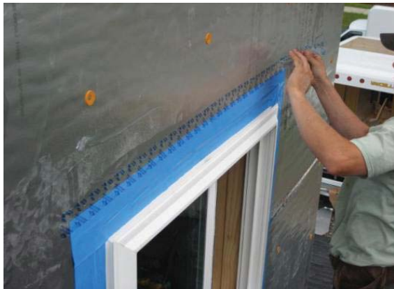
Flashing tape and weather resistant tape
