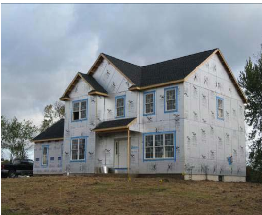
Exterior insulation and weather barrier tape
