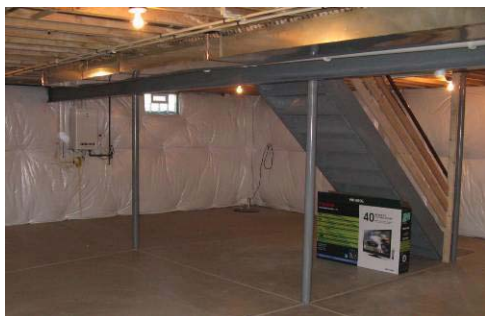
Basement Walls: R-25 fiberglass insulation blanket with perforated FSK facing
