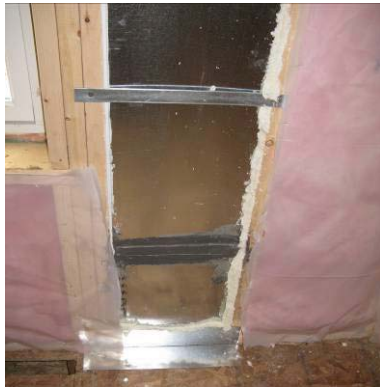
Wall cavity insulation and sealant
