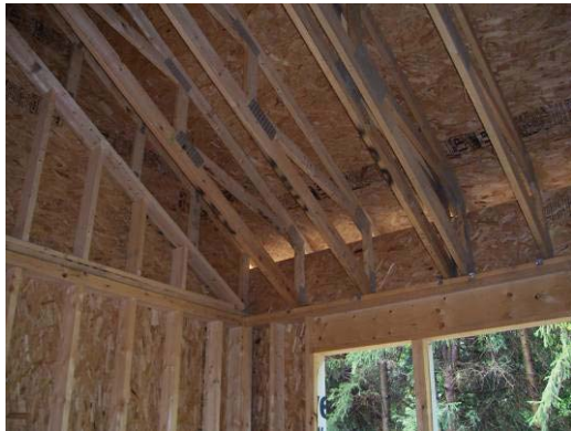
Ceiling and raised heel trusses
