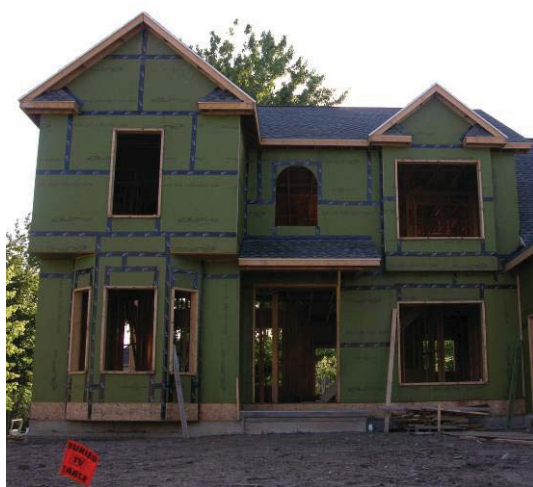
The Viola challenge home before attaching continuous foam insulation
