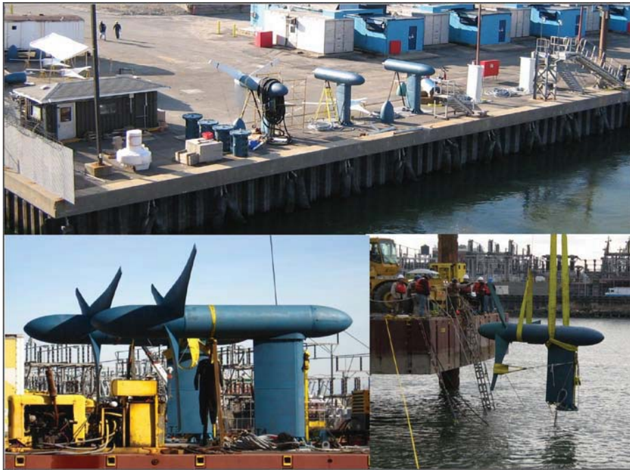
Fig. 6 – RITE Demonstration Deployment #2 - Turbine Assembly and Installation
