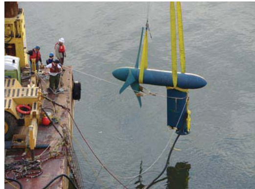
Fig. 5 – KHPS Turbine 1 (T1) Deployed December 11, 2006 (East River; New York, NY)
