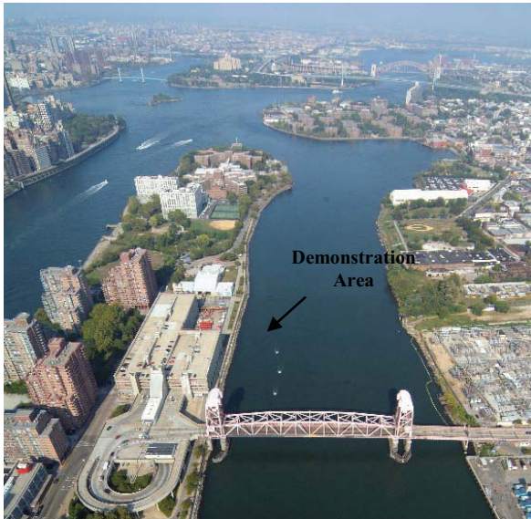
Fig. 3 - RITE Demonstration Site (Aerial View)
