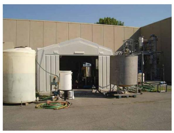
Figure 2-2. Picture of the Building, Influent Holding Tank and Anaerobic Influent Tanks
