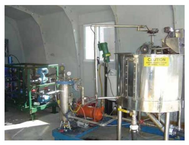
Figure 2-4. Recycled Flow Pressurization System – Krofta Supracell
