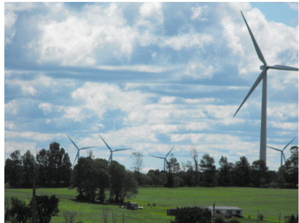
Wethersfield Wind Farm
