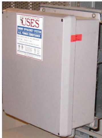
Figure 28. USES Case Detail Showing Security Screws and Tape Seal
