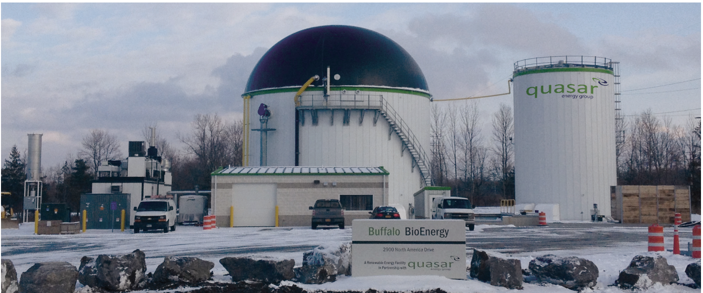
Buffalo BioEnergy Anaerobic Digester Gas, Erie County, NY
