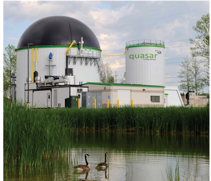
Buffalo BioEnergy Anaerobic Digester Gas, Erie County, NY
