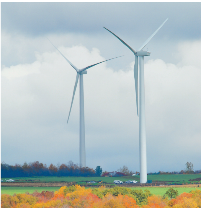
High Sheldon Wind Farm, Wyoming County, NY
