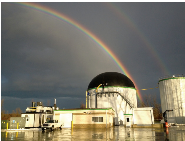
Buffalo BioEnergy Anaerobic Digester Gas, Erie County, NY
