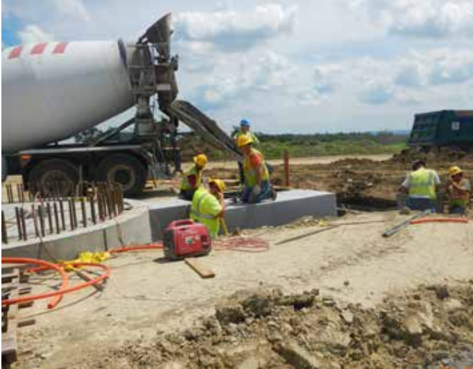
Construction of Orangeville Wind Farm, Wyoming County, NY
