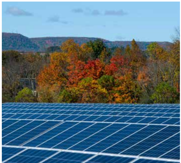
Owens Corning, Albany County, NY
