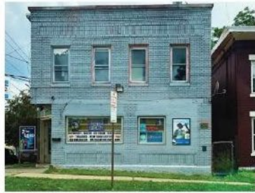
318 E Division St Onondaga County Year built: 1910 Units: 5
