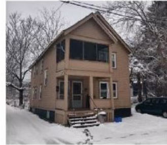
102 Lydell St Onondaga County Year built: 1900 Units: NA
