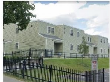
123 Livingston Ave Albany County Year built: 1985 Units: 200
