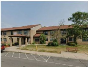
107 Trolley Barn Ln Onondaga County Year built: 1980 Units: 39
