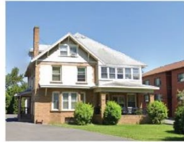
2111 E Genesee St Onondaga County Year built: 1900 Units: 6
