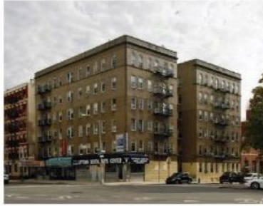
1 Audubon Ave New York County Year built: 1910 Units: 55
