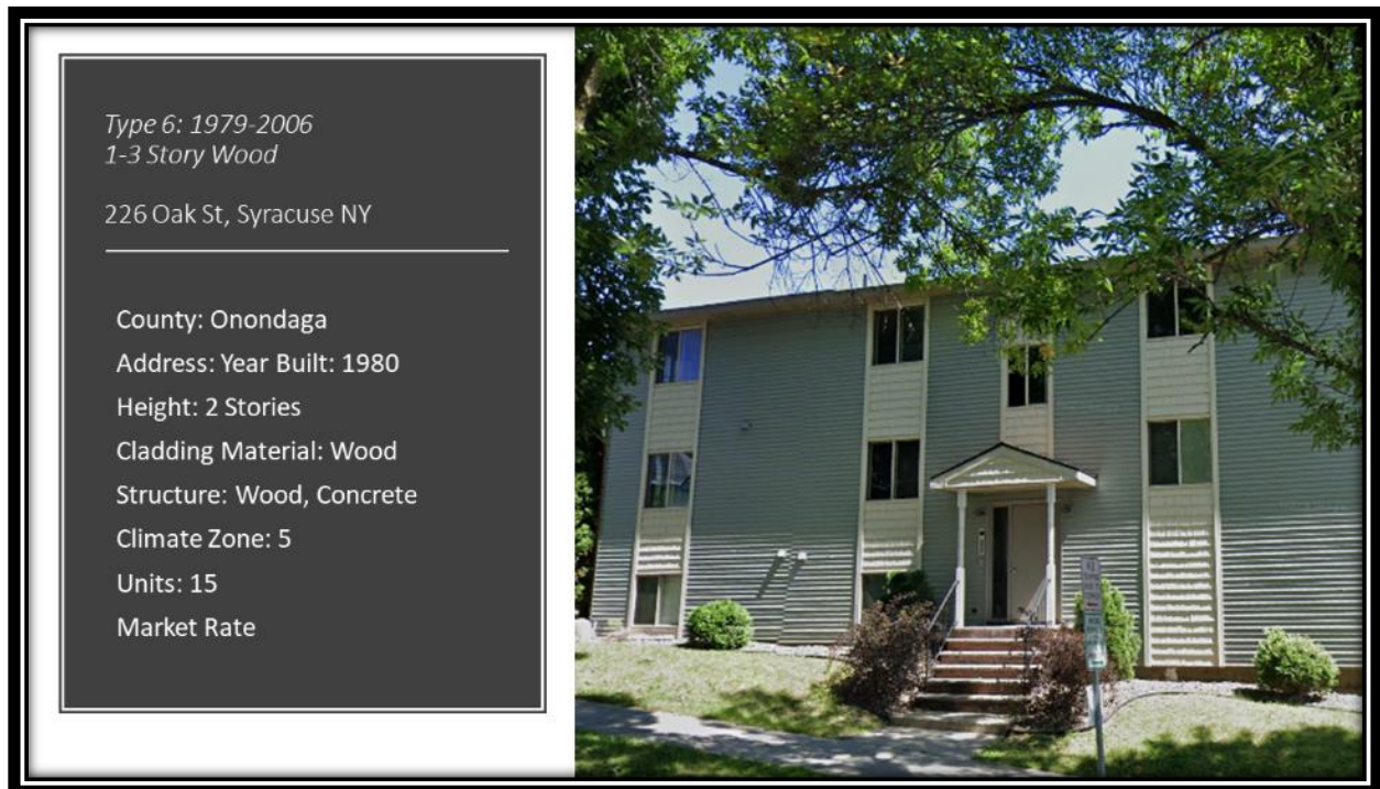
Figure 41. An Example of One- to Three-story Wood Frame Constructed Multifamily Housing from 1980
