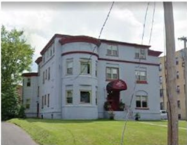
1114 E Genesee St Onondaga County Year built: 1890 Units: 10
