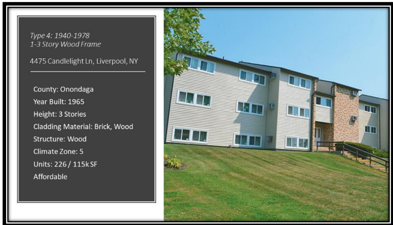
Figure 31. An Example of One- to Three-Story Wood Frame Constructed Multifamily Attached Housing from the Mid-1960s
