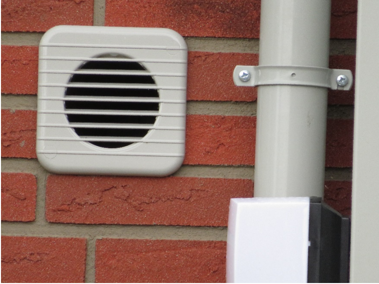
Figure 28. Room by room ventilation
