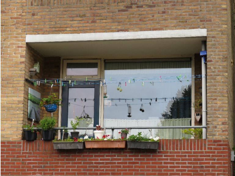
Figure A23. Recessed patio in building not yet renovated
