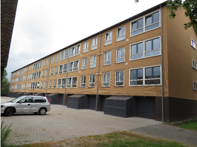
Figure A24. Renovated building
