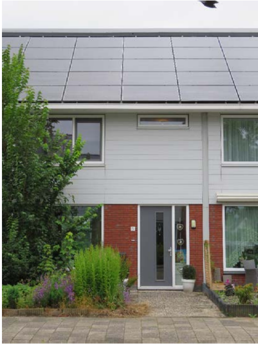
Figure A9 Front entrance/façade – solar modules on the roof
