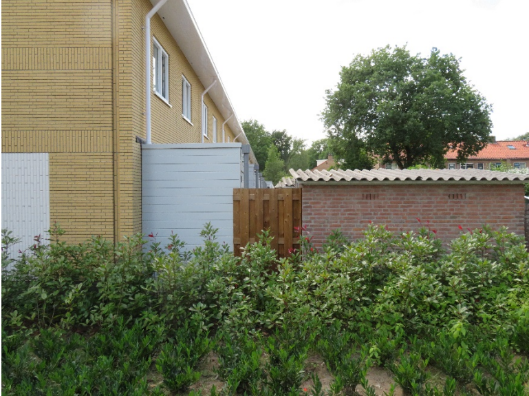
Figure A43. Mechanical sheds in rear of renovated building
