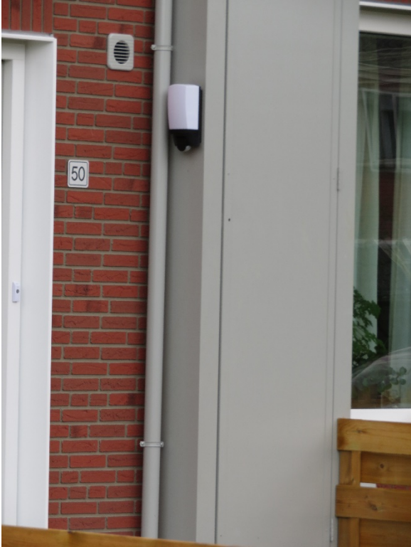
Figure 29. Exterior mechanical enclosure/chase
