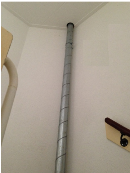
Figure 21. Exposed ductwork
