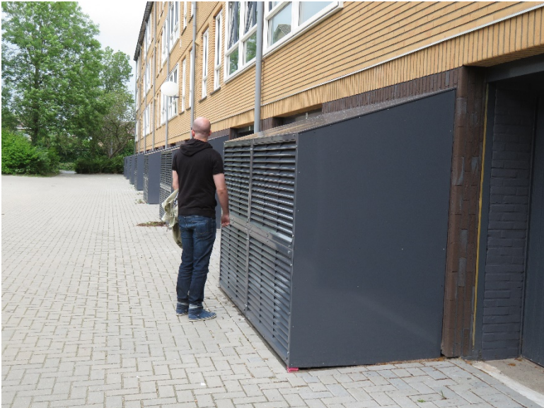
Figure A26. Exterior mechanical shed attached to renovated building
