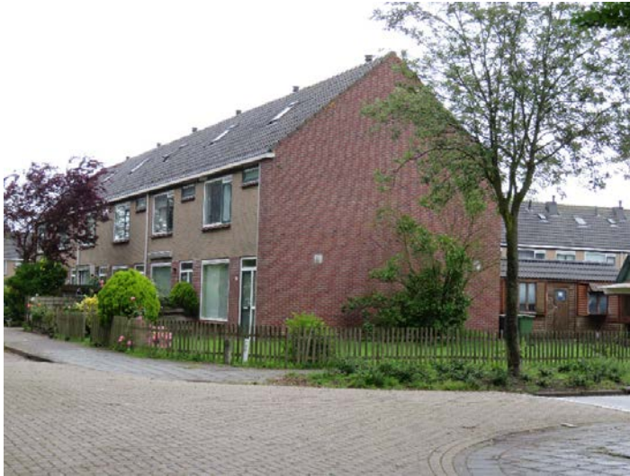
Figure A1. Building not yet renovated
