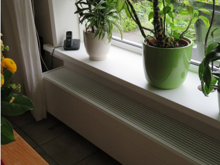
Figure A6. Radiator, below window extension used as a shelf
