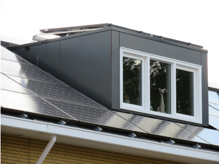
Figure A42. Dormer in renovated building
