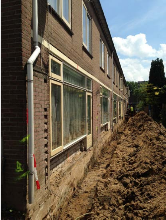
Figure A13. Excavation to add foundation insulation
