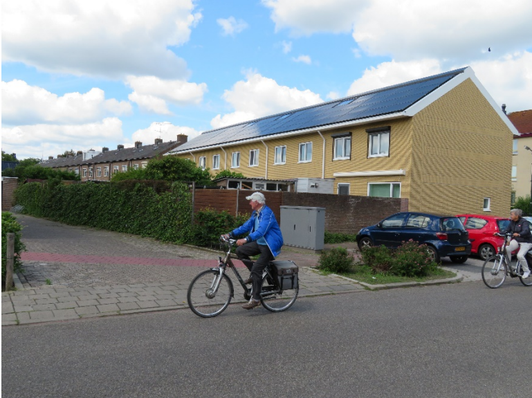
Figure A44. Renovated building
