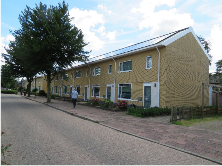
Figure A39. Renovated building
