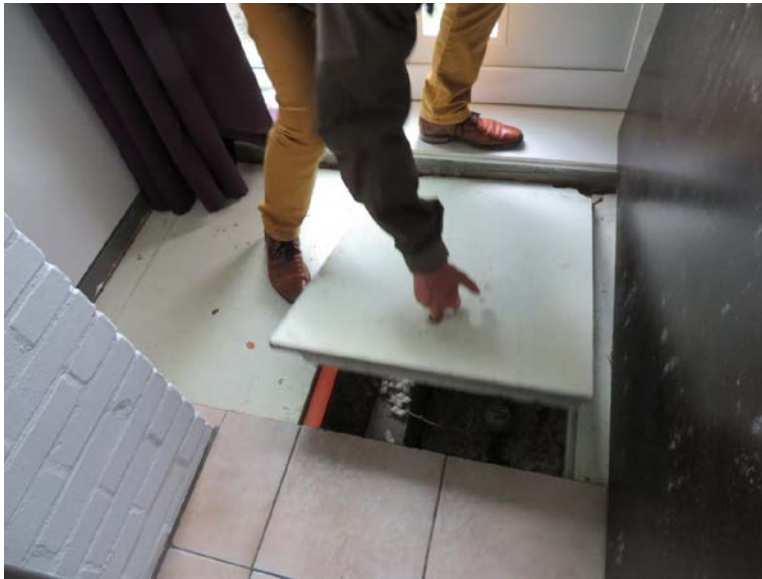
Figure 1. Floor panel access to crawlspace
