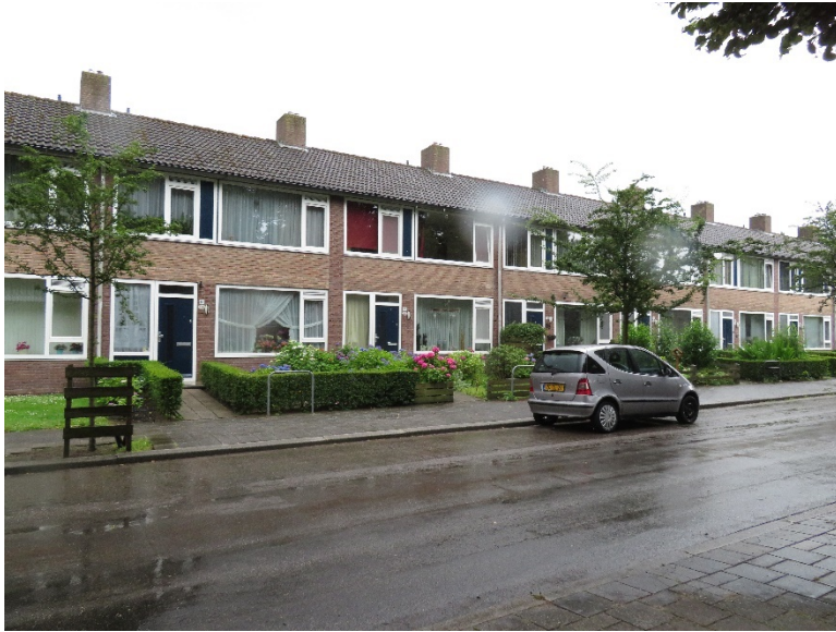
Figure A17. Building not yet renovated
