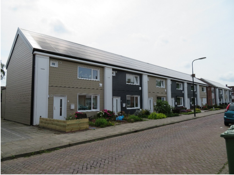
Figure A47. Renovated building
