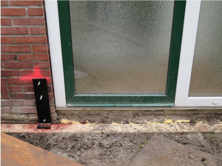
Figure 9. Structural fasteners attached to the wall
