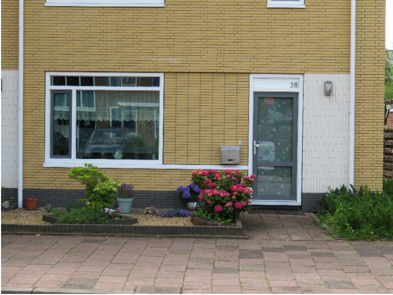
Figure A41. Renovated façade
