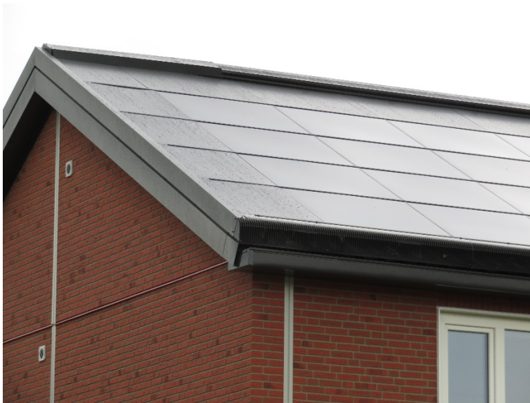
Figure 27. Roof-mounted heat pump heat exchanger: air grilles are above gutters and at roof peak
