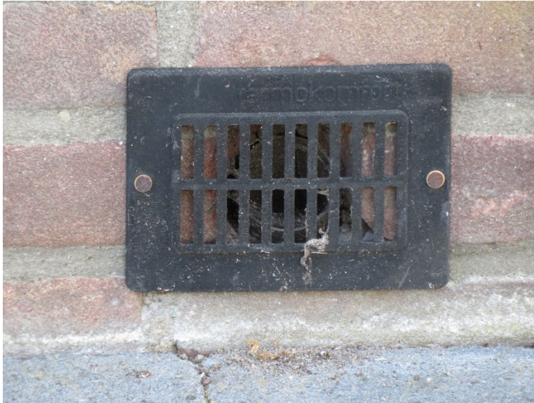
Figure A45. Crawlspace vent in not-yet-renovated building
