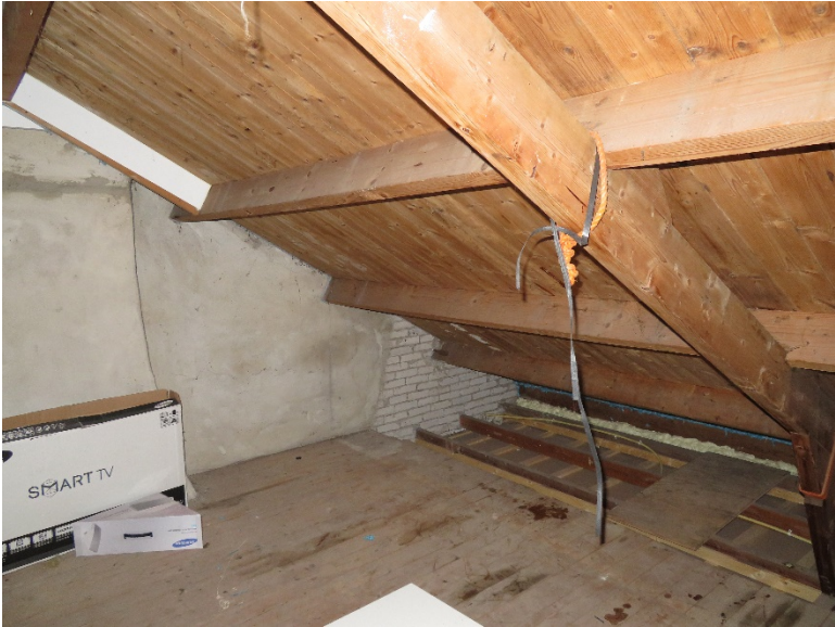
Figure A35. Attic in renovated building showing evidence of air sealing, but insulation is all exterior, above the roof-line
