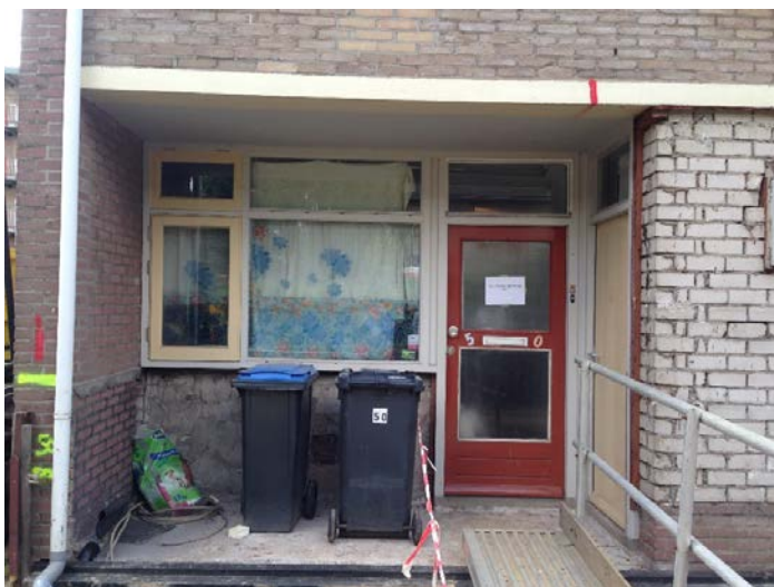
Figure A10. Pre-retrofit façade undergoing preparation for renovation
