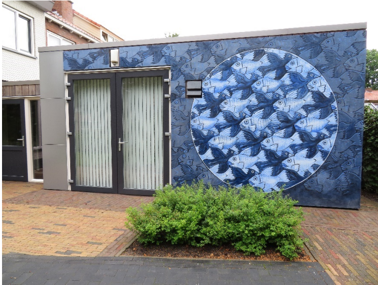
Figure 31. First floor “age-in-place” addition
