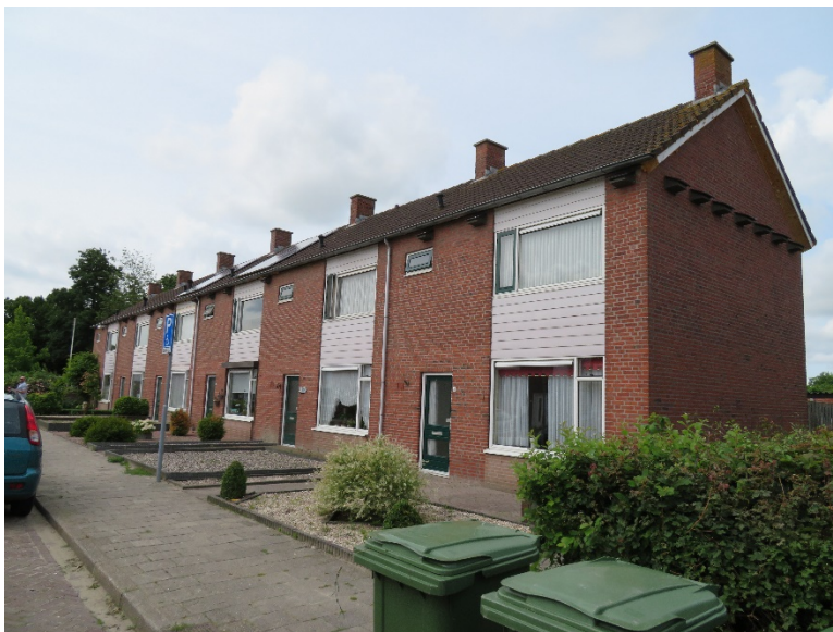
Figure A46. Building not yet renovated
