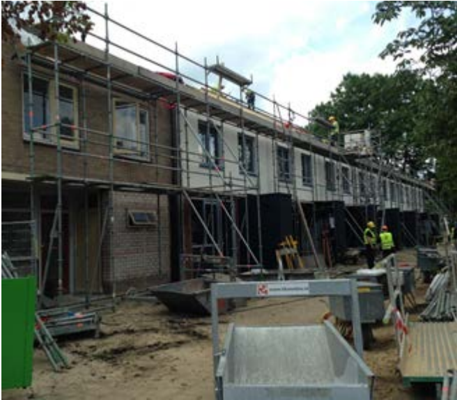
Figure A14. Existing façade and scaffolding for renovation
