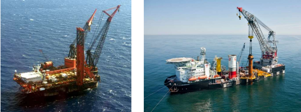
Figure 11.3-8 Heavy Lift Installation Vessel
