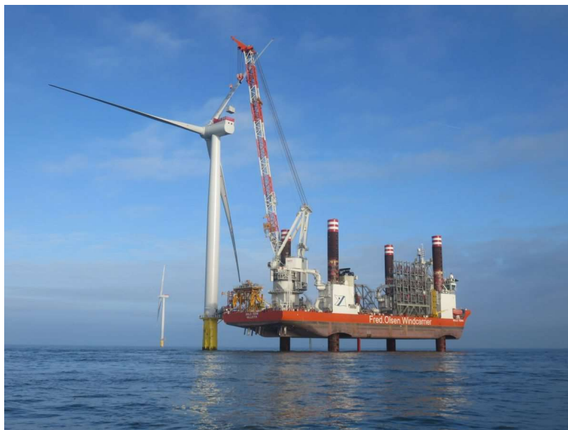
Figure 11.3-17 Turbine Installation Vessel
