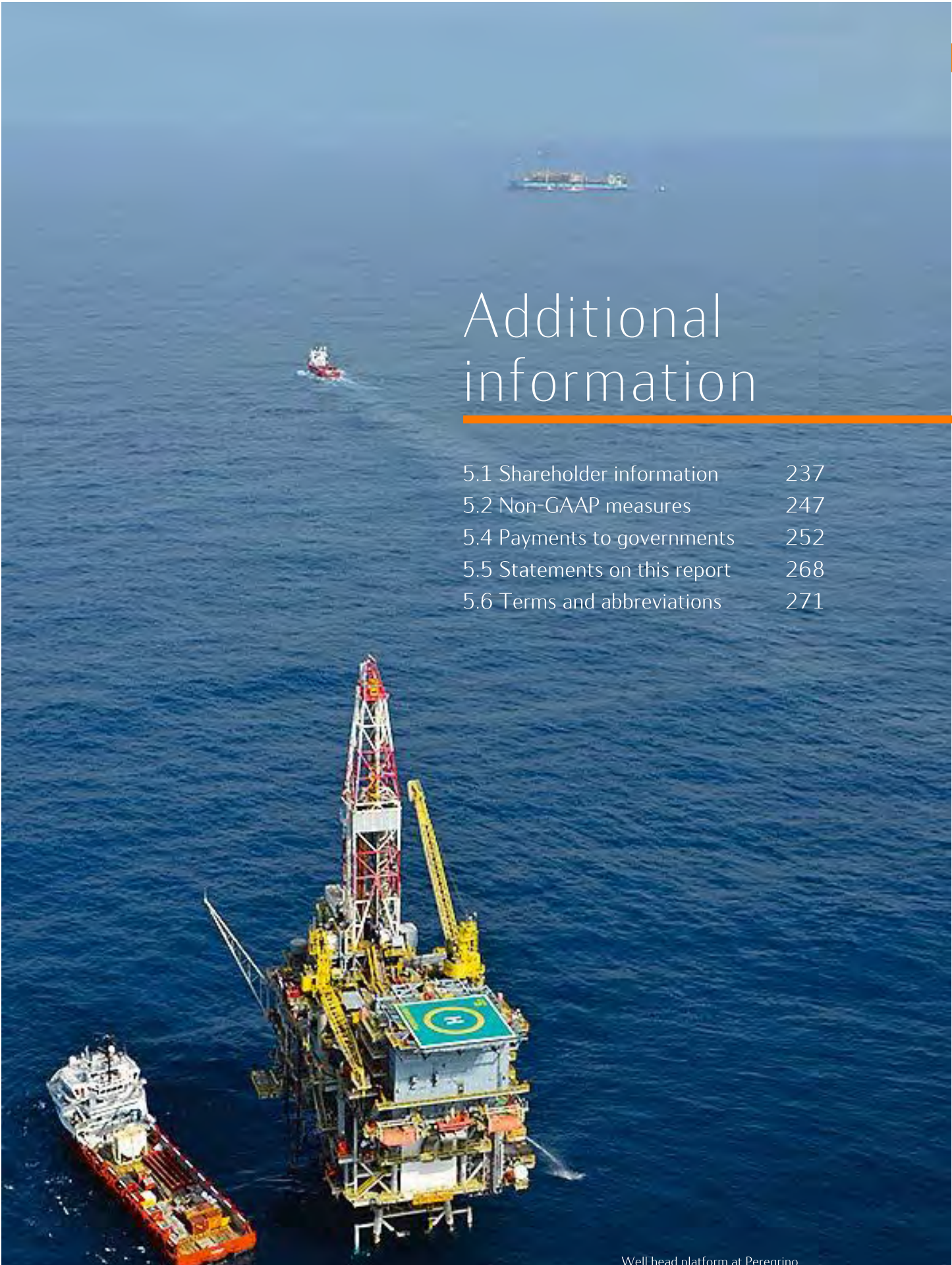
Well head platform at Peregrino.
