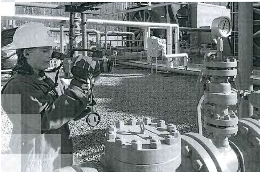
Shell is using infrared cameras to scan for methane emissions so that leaks can be repaired. Appalachia, Pennsylvania.
