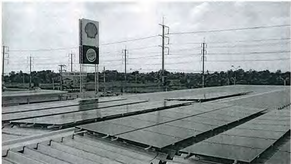
Solar panels are installed on the rooftop of a Shell service station in Thailand.
