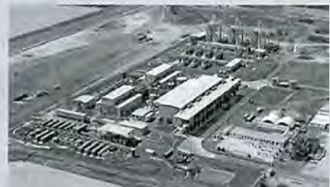
At the QGC Project, Australia, the central water treatment plant recycles salty underground water extracted during gas production.
