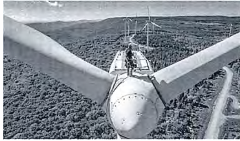
Our share of capacity from wind power projects is more than 400 megawatts.
