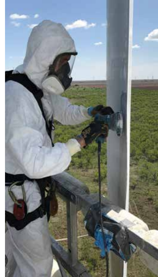
Repairing leading edge damage can increase AEP by as much as 20% .
