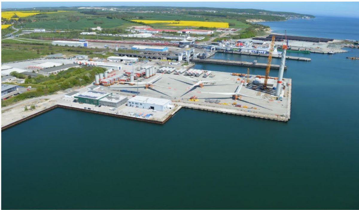
Figure 6-2 Arkona offshore wind farm in Sassnitz/Rügen
