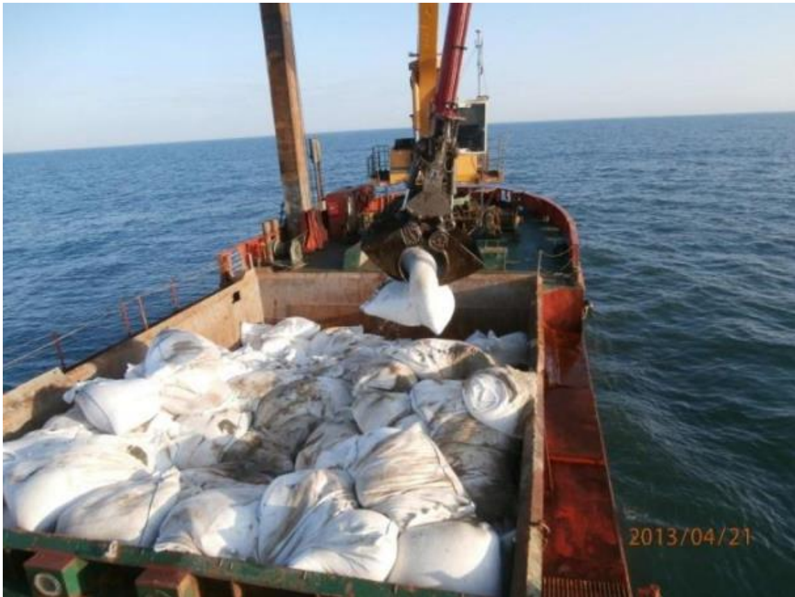
Figure 13-12 Example of sand container installation from RWE Amrumbank West wind farm, 2013
