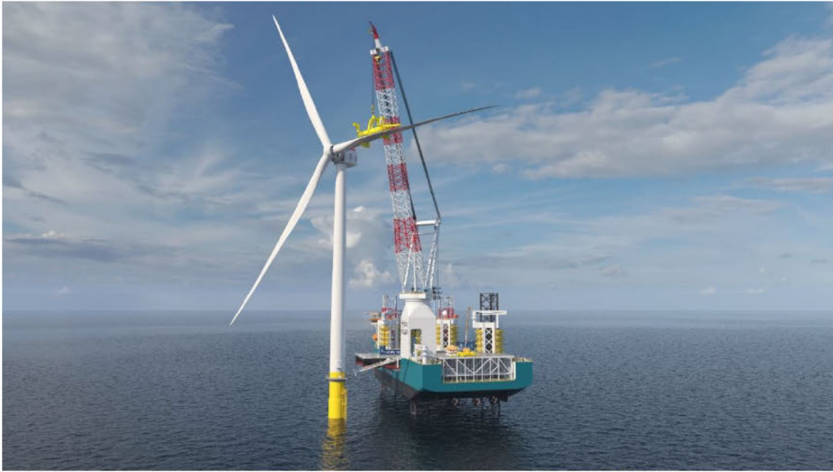
Figure 13-18 Havfram concept installing the blade using a jack-up vessel
