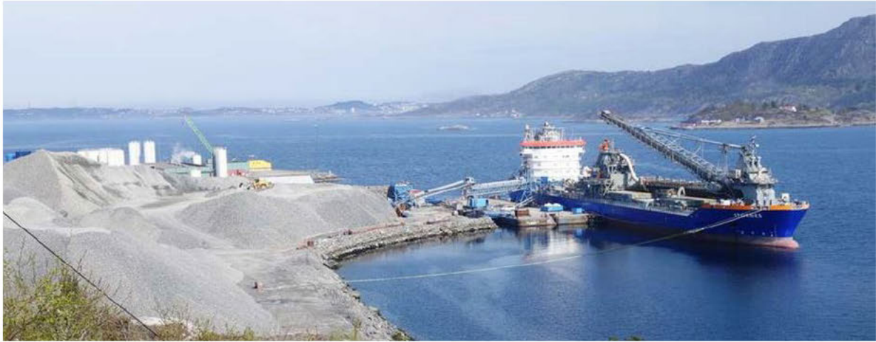
Figure 13-13 Example of loading rocks for scour protection
