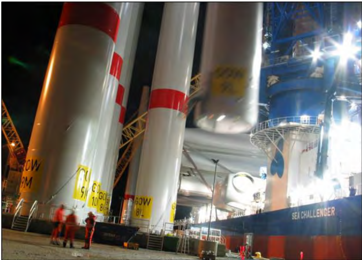
Figure 13.10 Loading Towers onto WTG Installation Vessel (Gode Wind, 2015)
