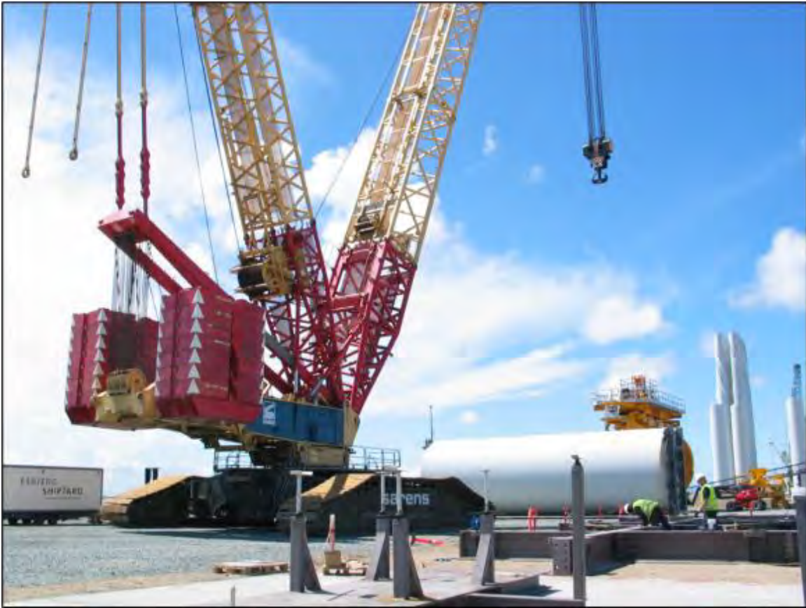
Figure 13.5 Upending of Tower Section in Load-Out Port (Gode Wind, 2015)
