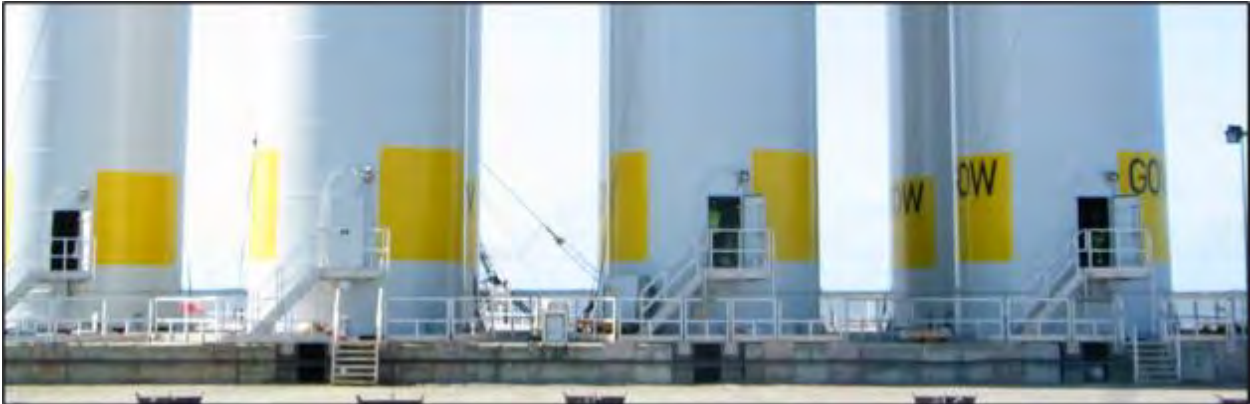
Figure 13.6 Towers Assembled and Ready at the Load-Out Port (Gode Wind, 2015)
