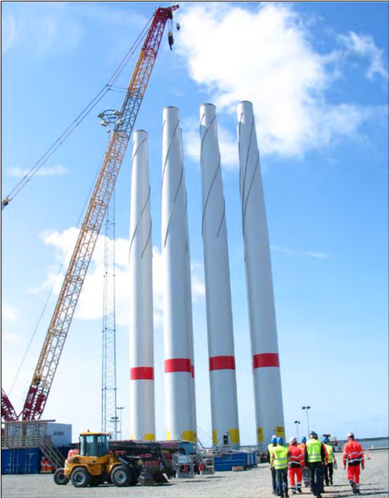
Figure 13.7 Towers Assembled and Ready for Load-Out (Gode Wind, 2015)
