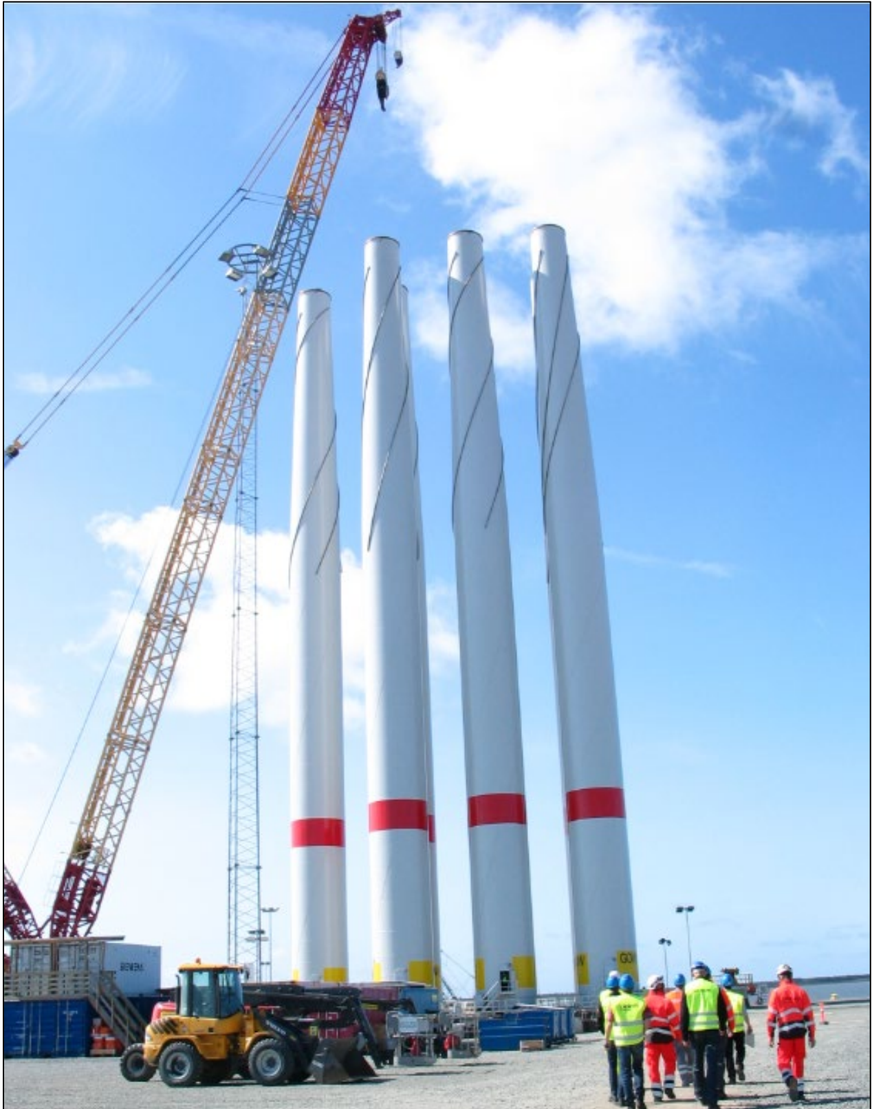
Figure 12.8 Towers Assembled and Ready for Load-out (Gode Wind, 2015)
