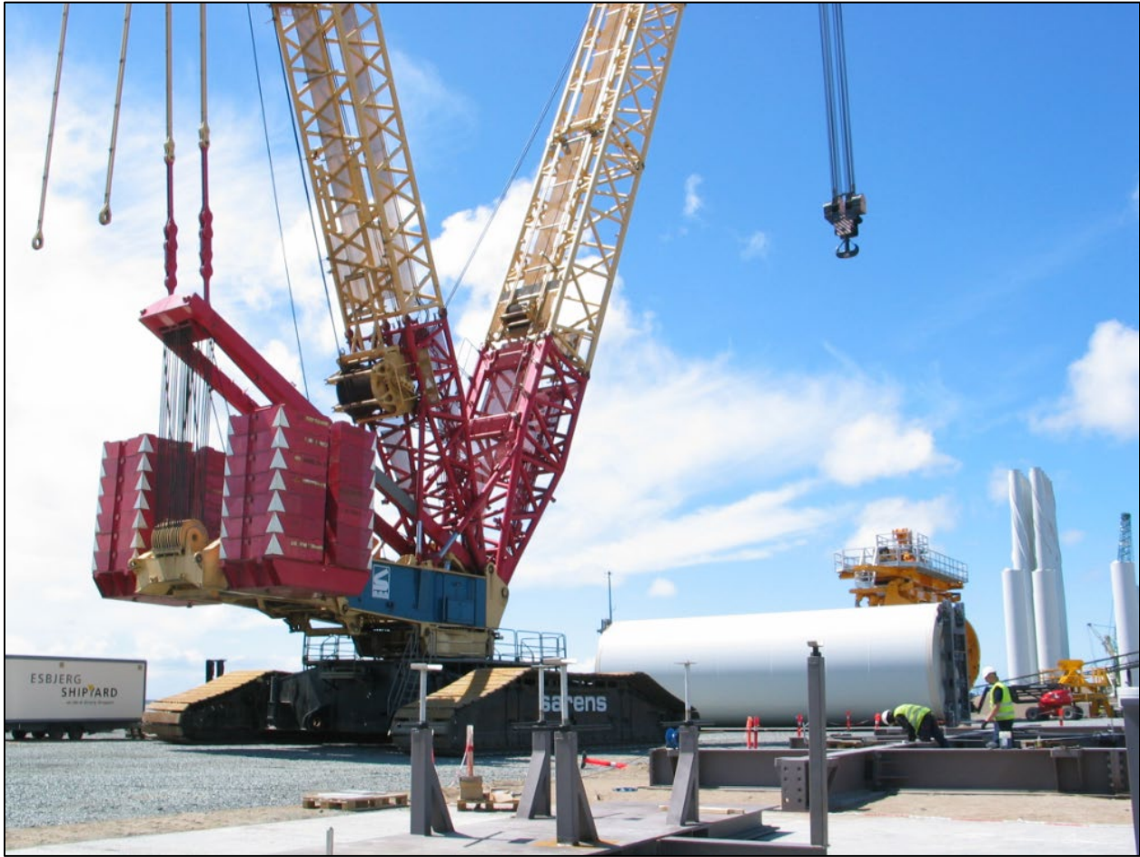
Figure 12.6 Upending of Tower Section in Load-out Port (Gode Wind, 2015)
