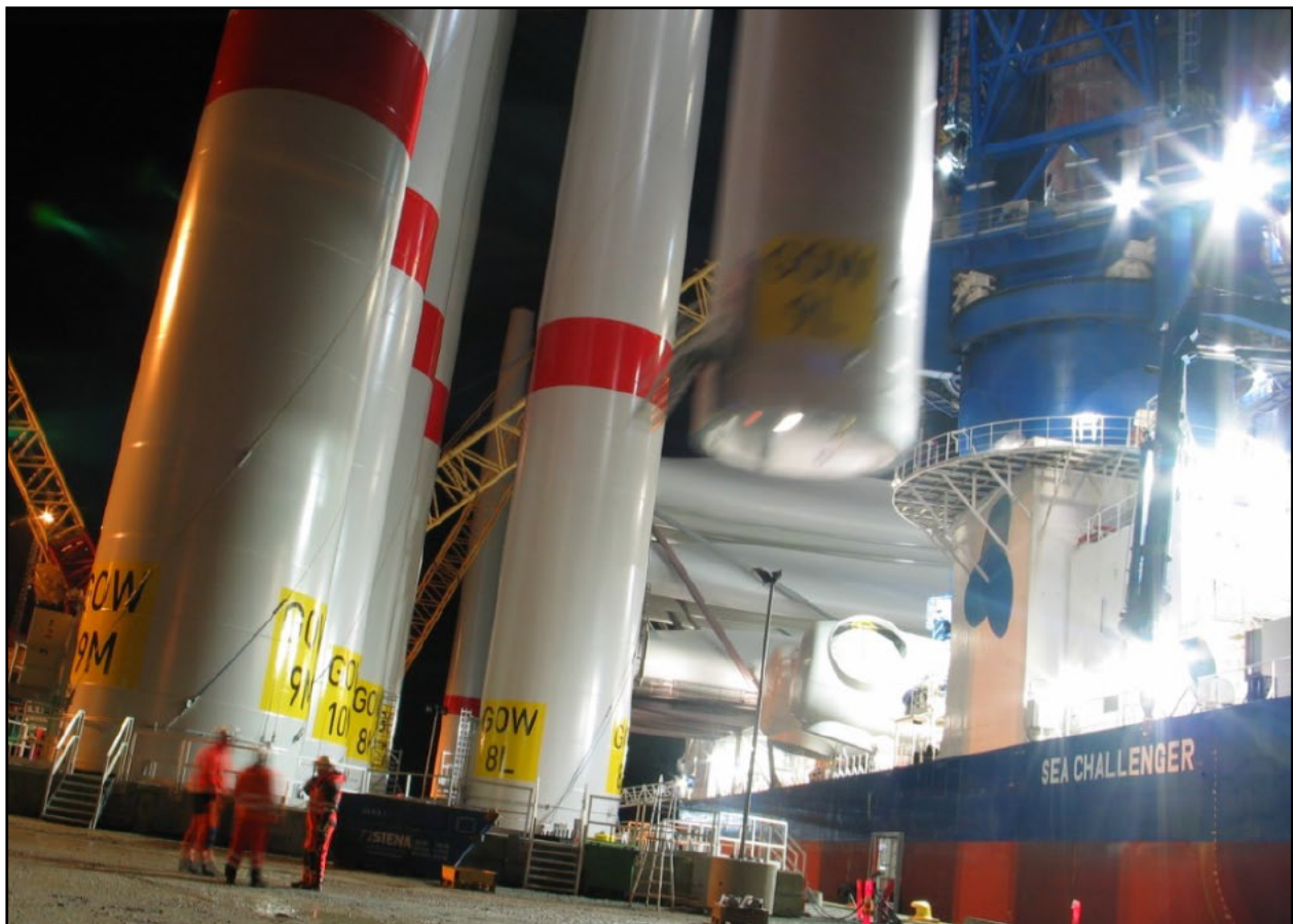
Figure 12.11 Loading Towers onto WTG Installation Vessel (Gode Wind, 2015)
