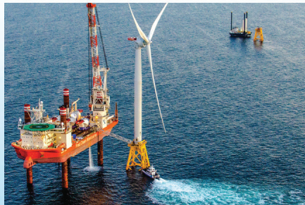
Wind Farm Construction
