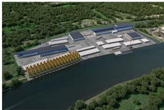
Port of Coeymans: Gravity Based Foundation Manufacturing
