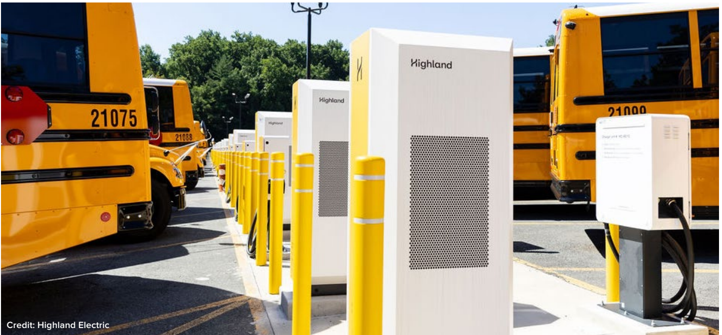
Figure 1: Charging Station with Bollard Protection
