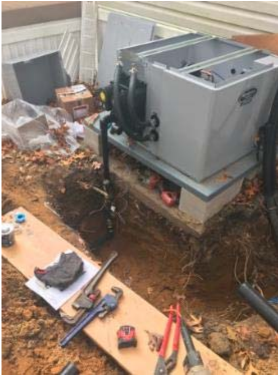
The outdoor split system at the Glenwood Village Site.
