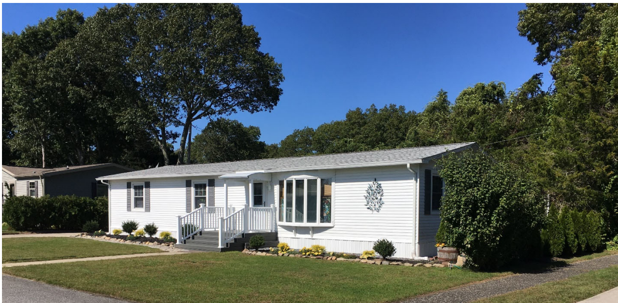
Figure 1. Photo of Typical House Installed on Ground Loop
