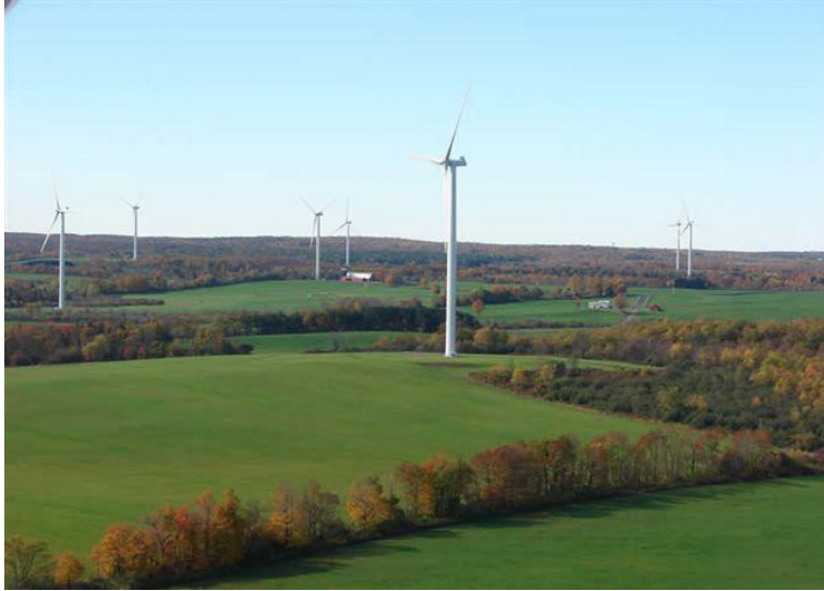
Maple Ridge Wind Farm, Lowville, New York
