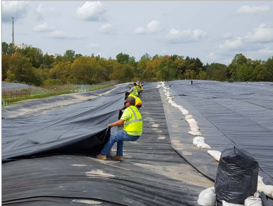
Figure 4-5. Sand placement and cap strap
