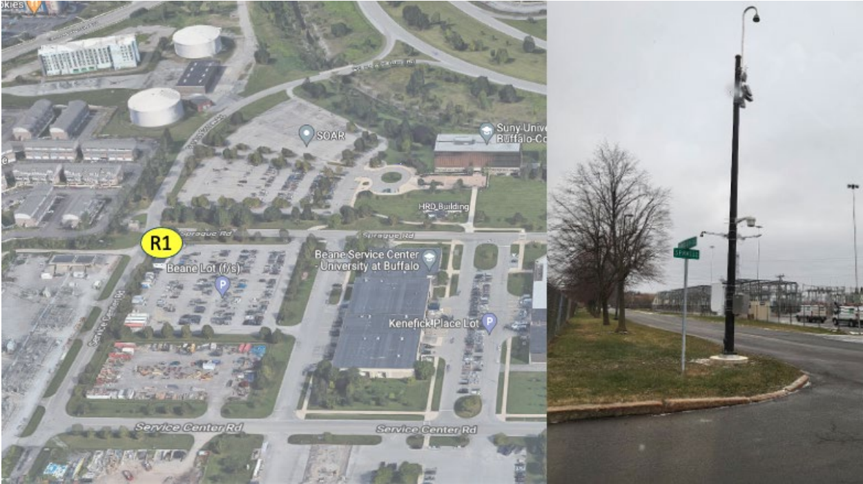
Figure 25. The Location Where RWIS is Installed on Service Center Rd, UB North Campus
