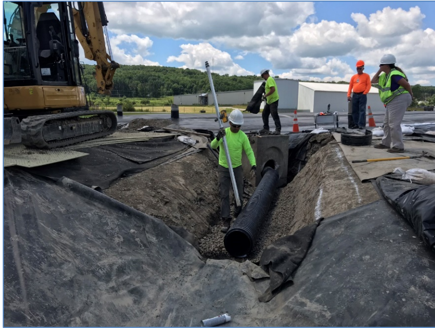
Figure 4-5. South detention basin completed work
