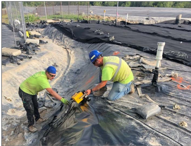
Figure 4-7. Geomembrane tie-in between the SDA and NDA.
