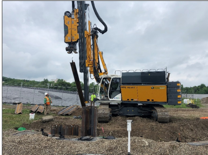
Figure 4-6. Steel-sheet pile installation.
