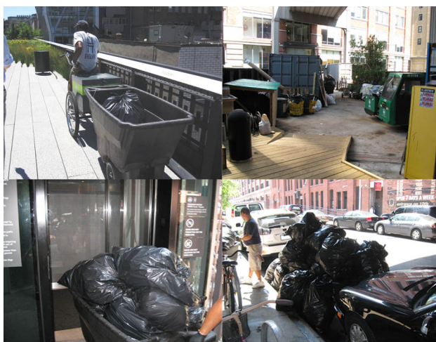
Figure 5-1. Current High Line Collection from Carts to Staging to Curbside (Via Elevator) (Source: Miller 2011)
