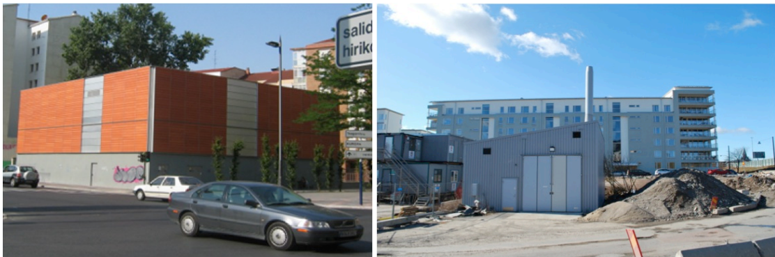
Figure 3-8. Temporary Terminals in Vitoria, Spain and Hammarby Sjostad, Sweden (Source: Envac, 2011)
