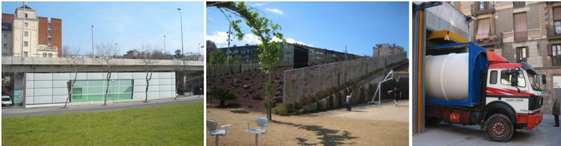
Figure 3-7. Terminal Installations Under a Bridge, Under a Park in Barcelona, and Under the Sub-Basement of the Santa Catarina Food Market in Barcelona (Source: Envac, 2011)
