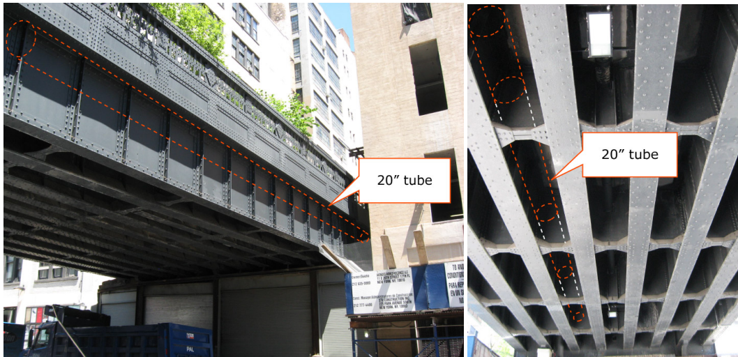
Figure 3-1. High Line, View From Street Showing Tube Location Along Side Or Between Girders
