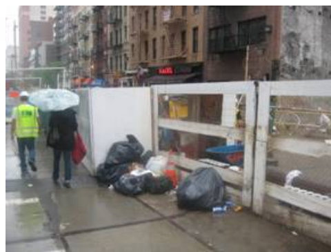
Figure 1-12. Second Avenue, on the Steel Plate Hanging Over a Cut-and-Cover Section (Source: Miller, 2012)
