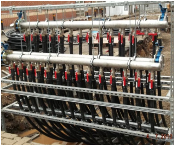
Figure 14. GLHE Manifold
