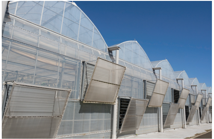
Greenhouse Ventilation Systems Inlets and Covers
