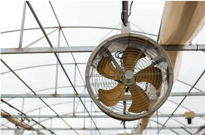
Horizontal Airflow (HAF) Circulation Fan System
