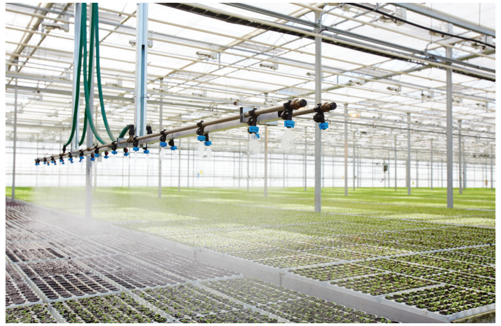
Greenhouse Fogging System for Cooling
