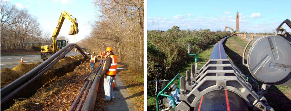
Figure 11.3-21 Neptune Project Installation Along Wantagh Parkway, Long Island
