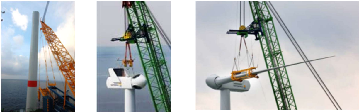
Figure 11.3-18 Installation of Tower Sections, Nacelle, and Blade
