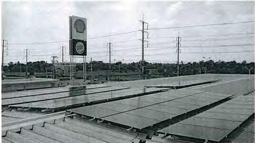
Solar panels are installed on the rooftop of a Shell service station in Thailand.
