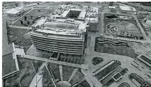
In 2017, we completed construction of our Shell Technology Centre Bangalore, India.
